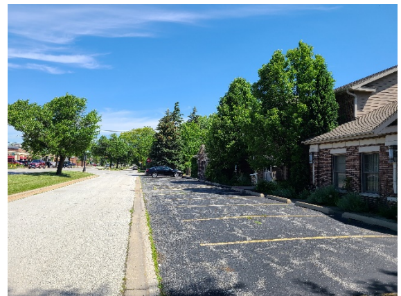
Looking North, Frontage Road & Parking Spaces
