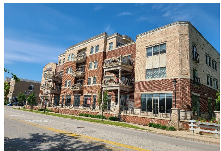
Existing Front Facade
